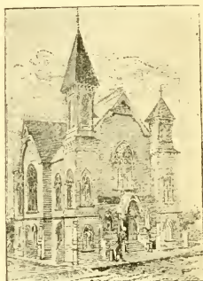
HOMER ST. METHODIST CHURCH, VANCOUVER.
